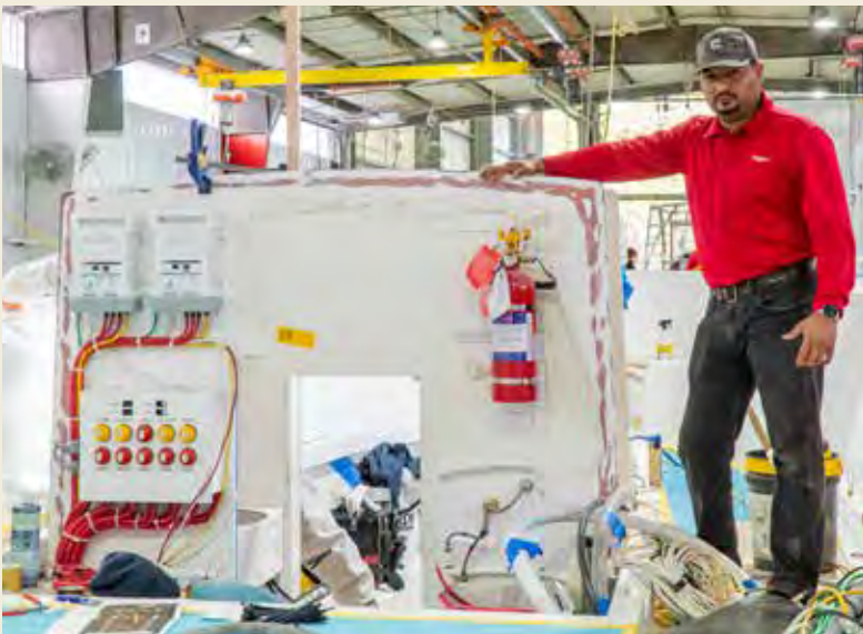
Foreman Melvin Bonilla overseeing V-46 mechanical installations.
