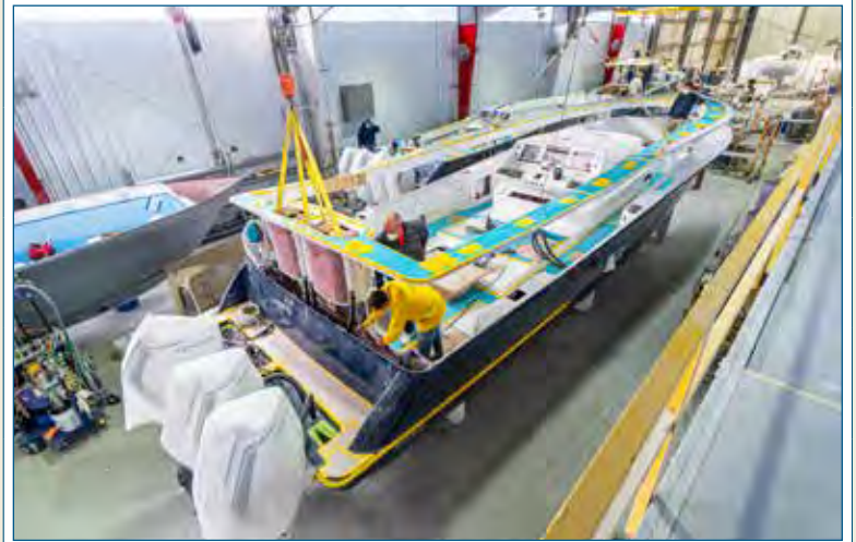
The coaming (with rod holders and transom live wells) is lowered into position.
