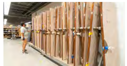
Interior doors are first hung by the Carpentry Department, and then removed and stored in a protected area before final installation by Exterior Trim.
